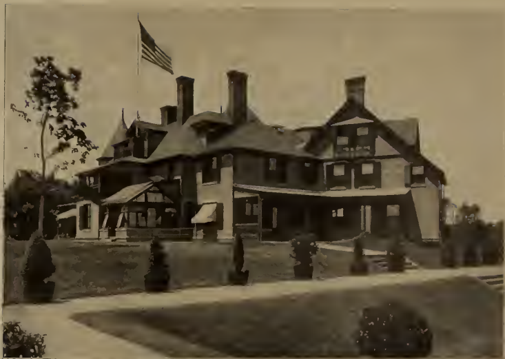
"BLETWAYDIN" RESIDENCE OF FRANCIS BLAKE, Worcester, Mass. 1898.
